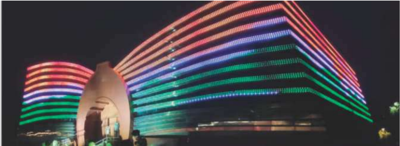
Hon'ble PM Shri Narendra Modi laid the foundation of one of the significant places in Panchteerth-Dr. Ambedkar National memorial, on 21/03/2016.
